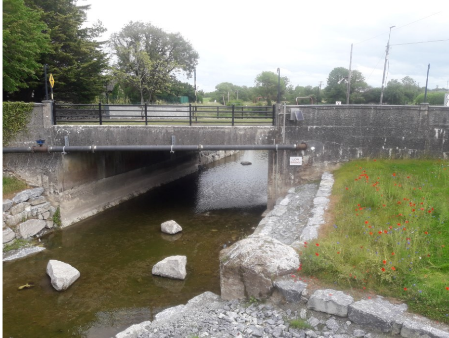
Figure 8: Regrading of Dunkellin complete
